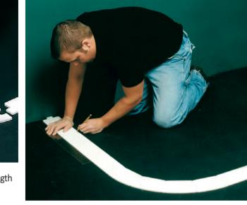
Layout Cards simply snap together to represent the exact length and shape of the assembled Glass Block design to act as an instant template for any design.
