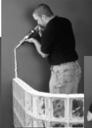
Place the second panel on top of the first and push into the wall until the vertical joints line up. (Tip...if the second panel is hitting the anchor at the wall and the vertical joints don't line up; pry the first panel out away from the wall until they do.)
