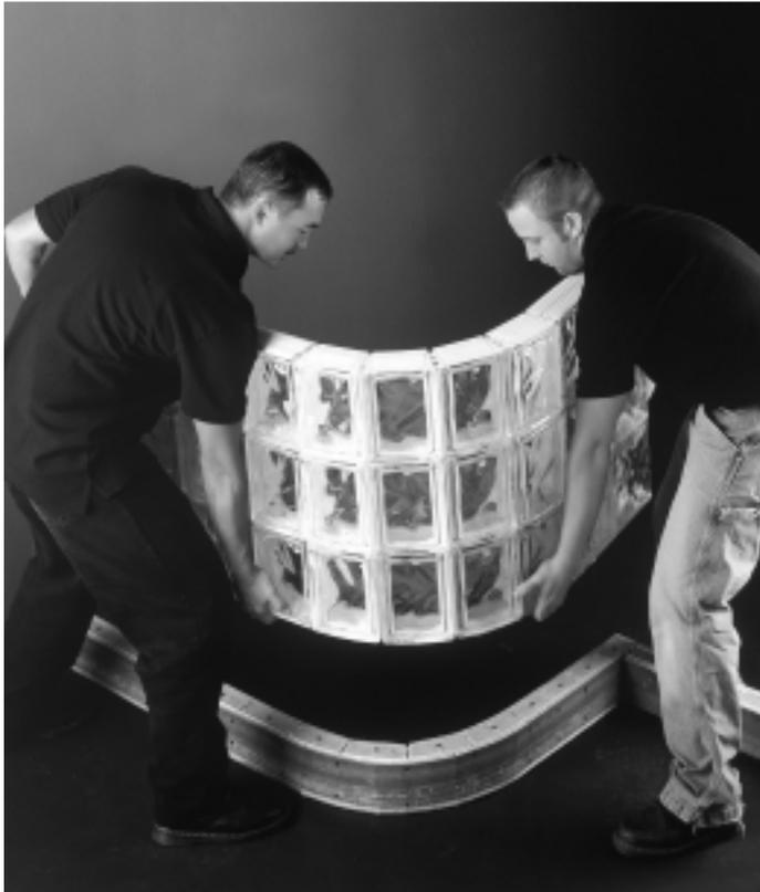
Plumb and level panel and drive a screw through upper hole of anchor. If anchoring through stone or tile, predrill with a 5/32" masonry bit. Once the first screw is in place, check your panel again for plumb, if a small adjustment is needed, the panel can be moved, and will pivot on the upper screw. When perfectly plumb, anchor with second lower screw.
