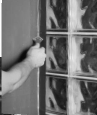
When desired finish of sealant is accomplished remove the tape on both sides of your fresh sealant pulling the tape at 45 degrees to the panel so that it doesn't disturb the sealant. Once the tape has been pulled, spray one more time and run your finger over the joint once more, this will smooth out any imperfections left by the removal of the tape.
