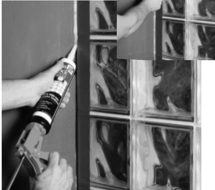
When desired finish of sealant is accomplished remove the tape on both sides of your fresh sealant pulling the tape at 45 degrees to the panel so that it doesn't disturb the sealant. Once the tape has been pulled, spray one more time and run your finger over the joint once more, this will smooth out any imperfections left by the removal of the tape.
